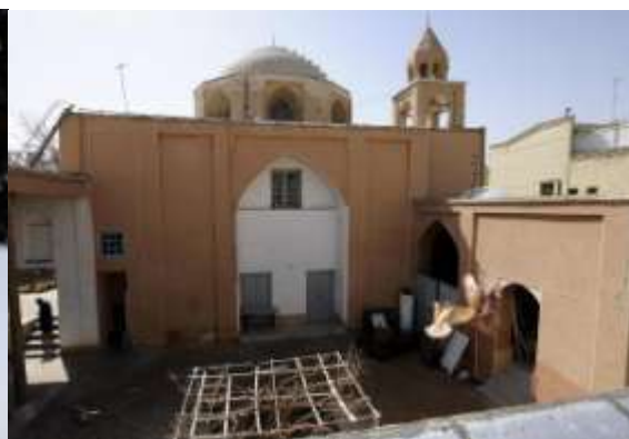
Figure 8. St. Nicholas church (exterior view)
